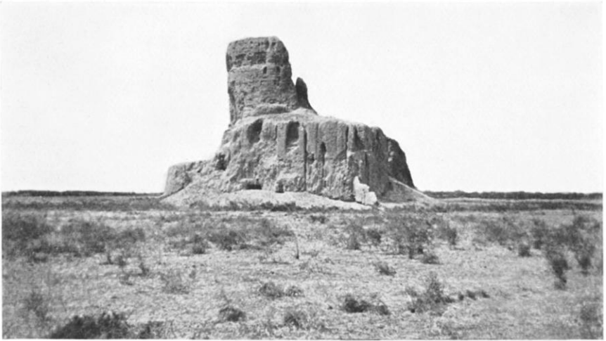
Ruined building in Balkh
